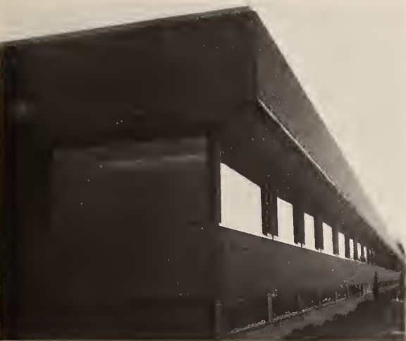
Wing "D" was added to the old academic building during the summer of 1966 in order to provide necessary lab space and offices for expanding teaching staff.
