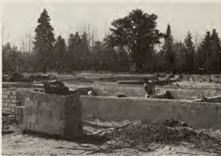
Construction on the new Residence Building began with the spring thaw.
