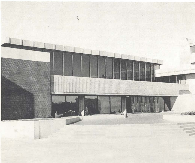
CENTENNIAL BUILDING AGORA ENTRANCE
